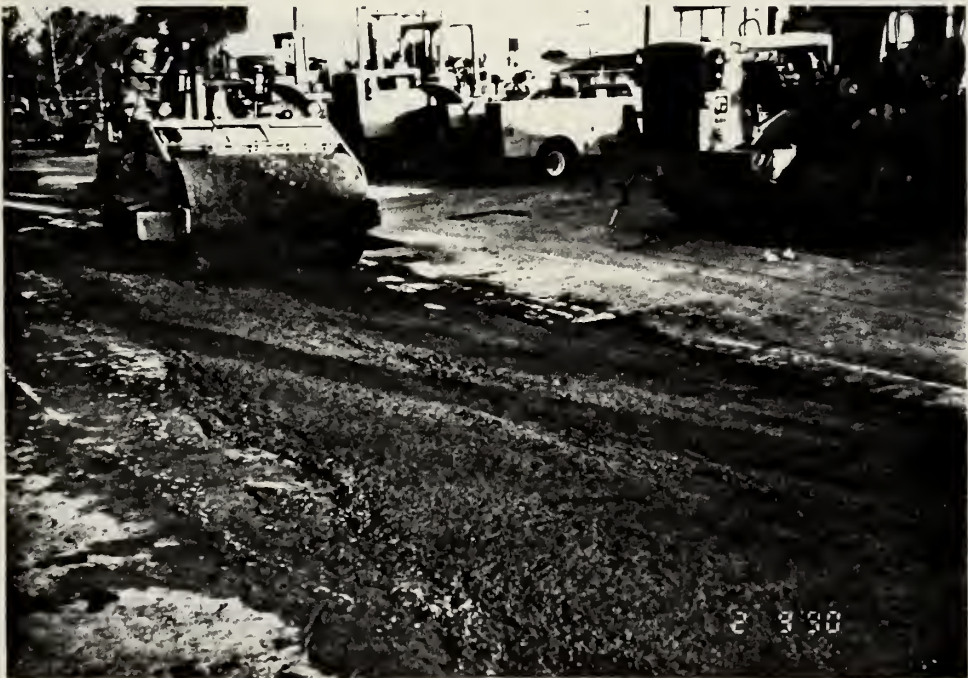
Figure 2.22 Vibratory Roller and Entire Slab View
